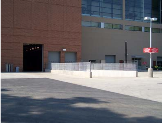
Outside loading area
